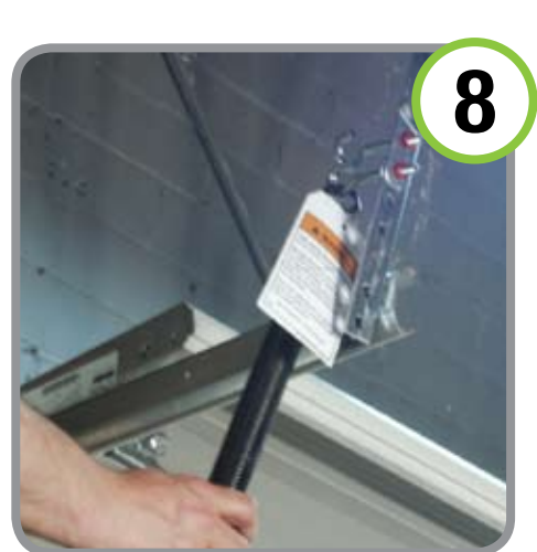
Remove spring from it's rear attachment point.
