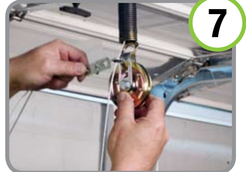
Thread cable through clevis pulley
