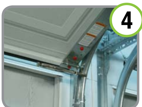
Place clamps, or locking pliers on the track, under BOTH bottom rollers.
